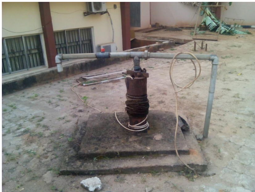
Figure 6: BOREHOLE HEAD AT PERM. SITE
