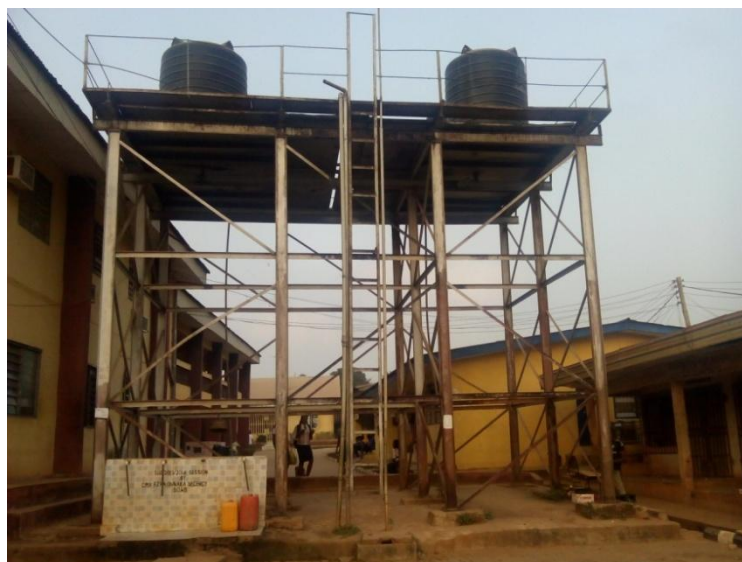
Figure 3: OVER-HEAD TANK AT THE TEMPOARY SITE
