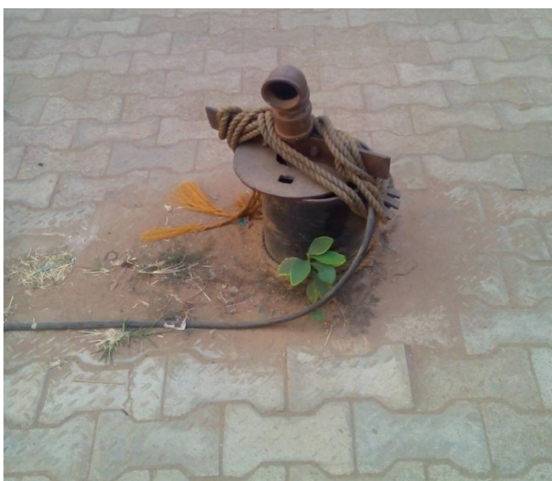
Figure 4: BOREHOLE HEAD
